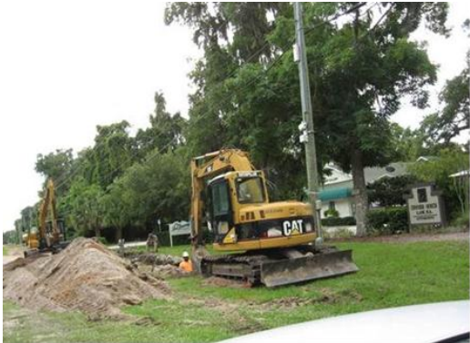
Installation of 8" PVC Pipe on A1A
