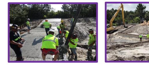
Start date of 2-18-13 for a 6 month contract time. All concrete completed for all structure caps. Started preliminary grading and rip rap installation. Working on formwork of the bulkhead caps. Preliminary electrical service and controller installation is underway. Site is experiencing dewatering issues and delays due to recent rain, however production continues. Project is 85% complete
