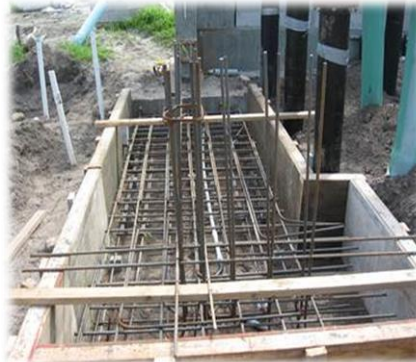
North Side Wall Footer
