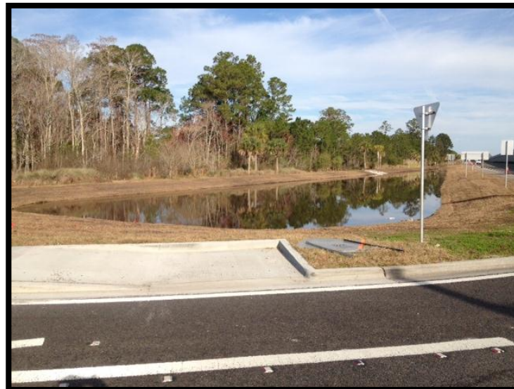
Finished Pond – Northwest Quadrant
