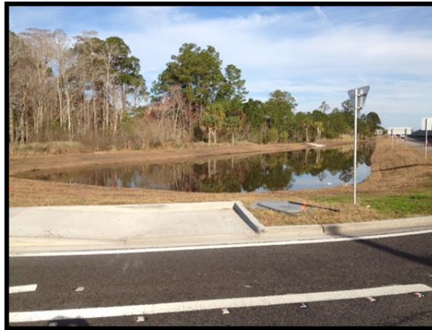
Finished Pond – Northwest Quadrant
