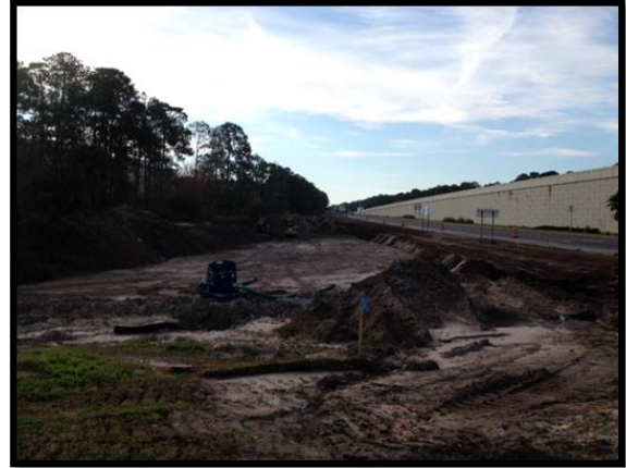
Construction – Southeast Quadrant
