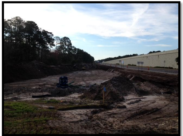
Construction – Southeast Quadrant
