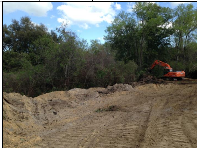
CLEARING WORK BEING DONE @ HOLLAND PARK
