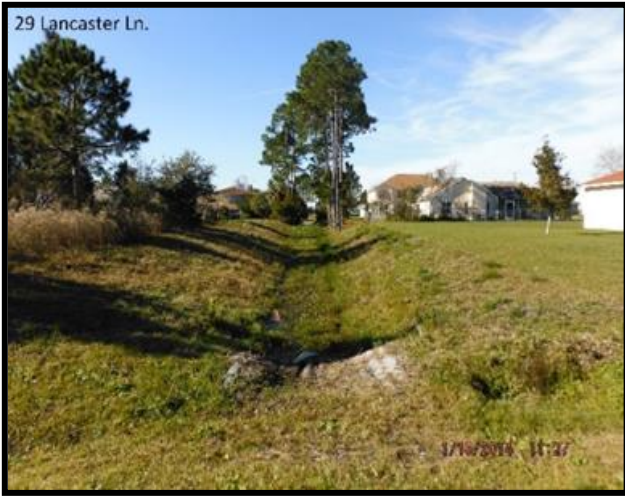
“BEFORE” – STORMWATER MODELING CONSTRUCTION SEC. 37 TRIBUTARY 2
