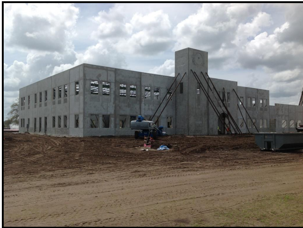
PALM COAST CITY HALL UNDER CONSTRUCTION
