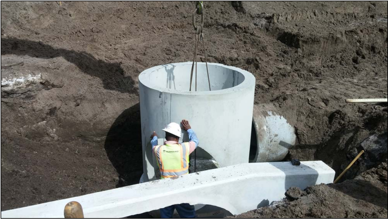
Palm Harbor Stormwater Head Wall on Forest Grove
