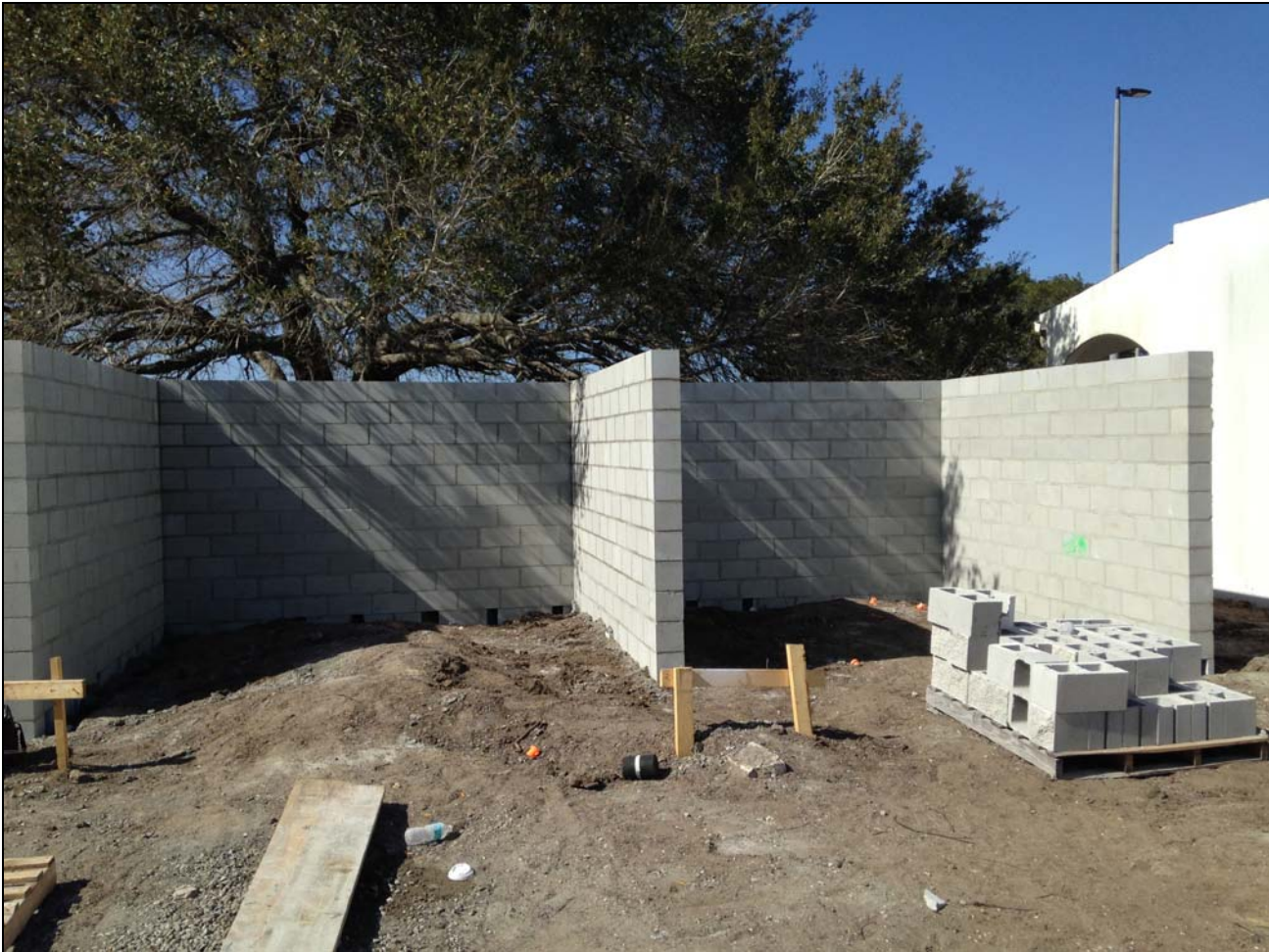
Holland Park Material Storage Bin
