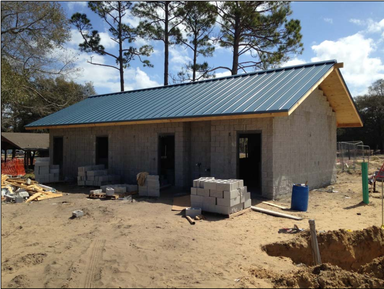
Holland Park Restroom
