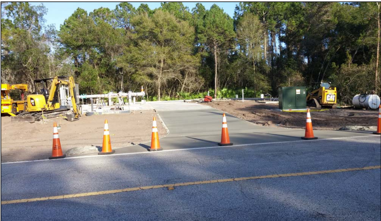
Old Kings Road Master Pump Station Driveway
