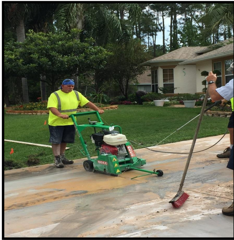
Driveway replacement for Swale Rehab on Brushwood Lane
