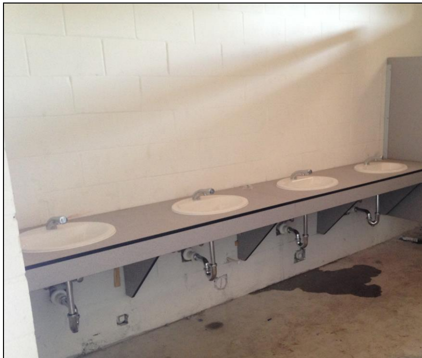
Bathroom Renovations @ Holland Park
