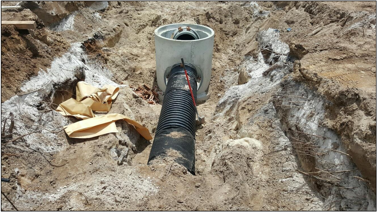
Tractor Supply - Storm Water Pipe Installation
