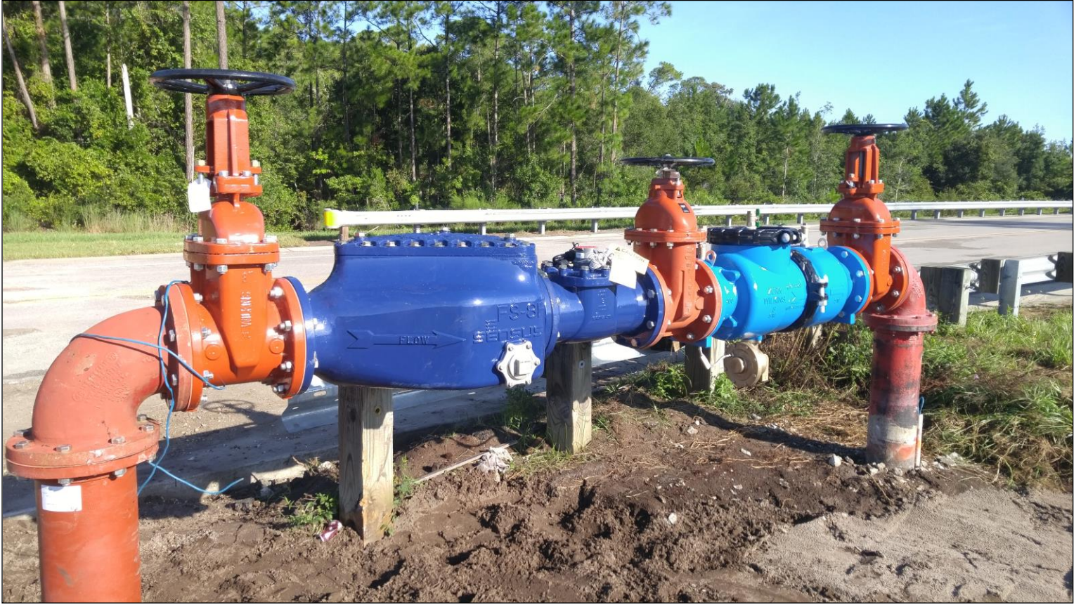
Airport Access Road - 8" Meter and Backflow Installation
