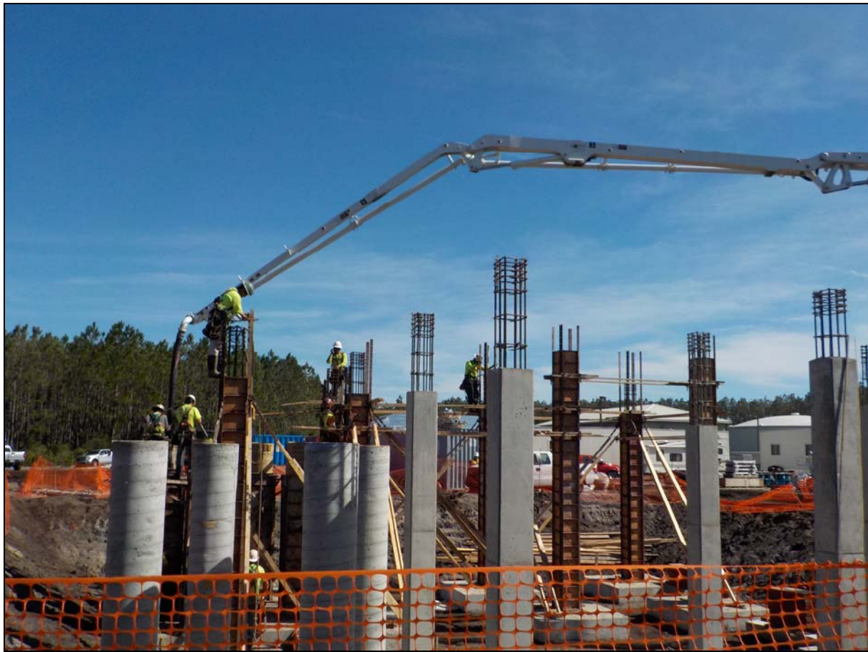
Waste Water Treatment Plant 2 – Concrete Placed in Headworks
