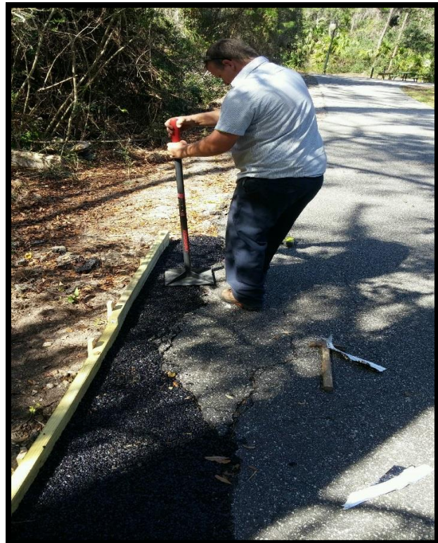
St. Joe's Trail Asphalt Repair
