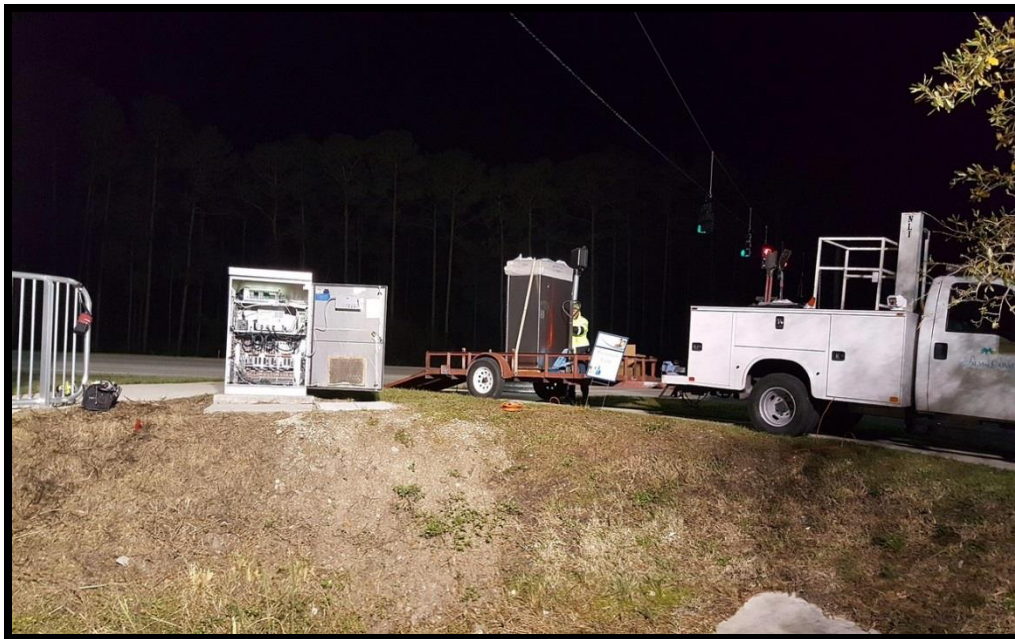
Late Night Traffic Cabinet Replacement
