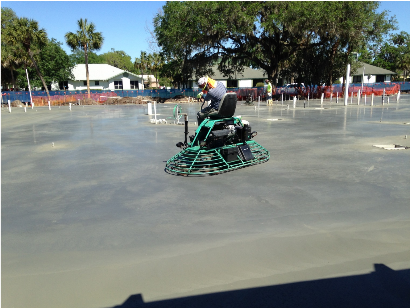
Community Center - Concrete Slab Finishing
