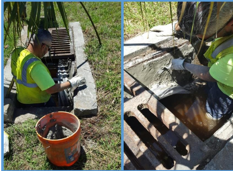
Catch Basin Repairs - Universal Trail
