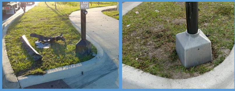
Pedestrian Pole Damage Repair - Cypress Point Parkway & Palm Coast Pkwy
