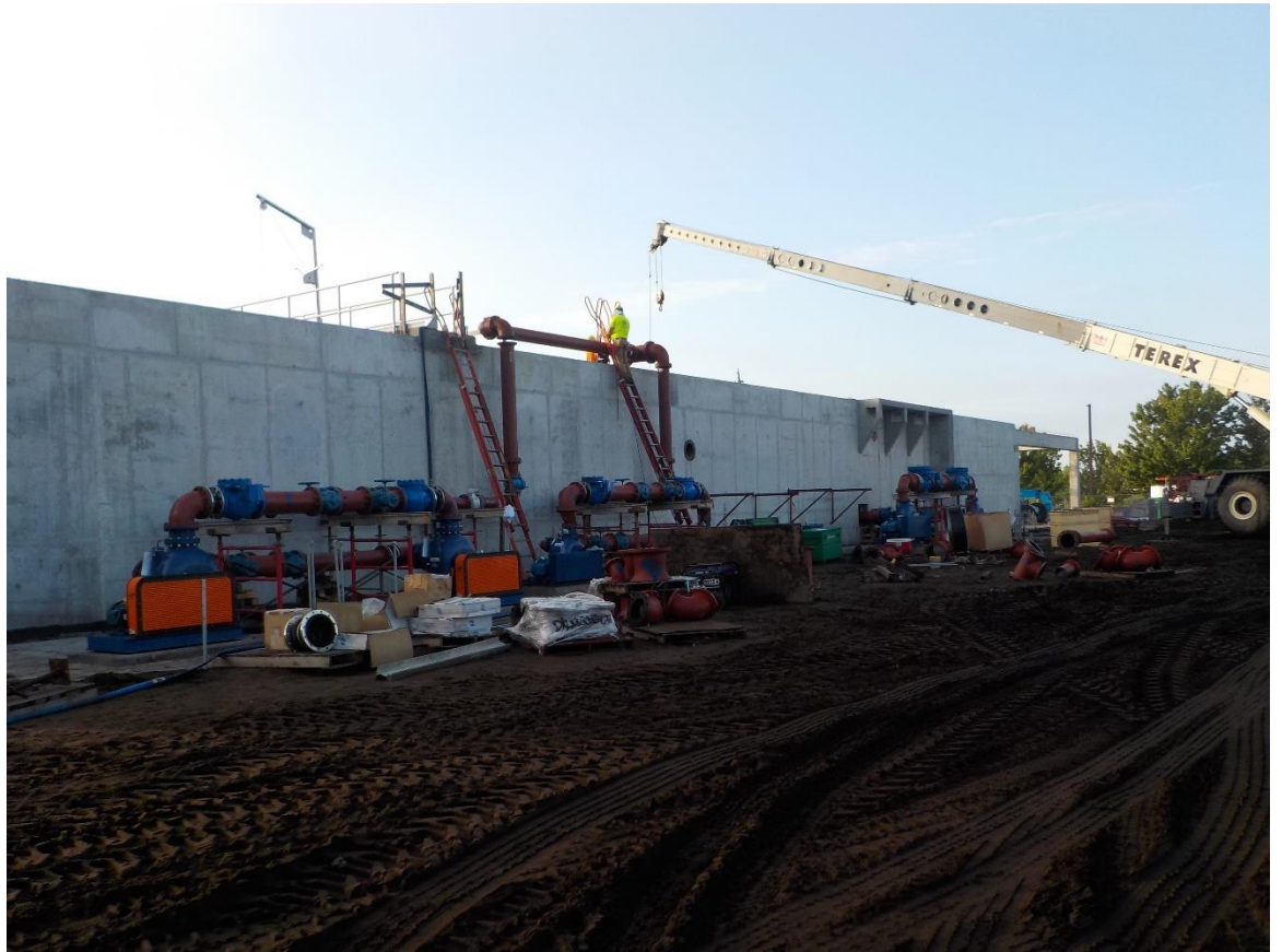
Waste Water Treatment Plant 2 – Pumps and Blowers for Biological Process Tanks
