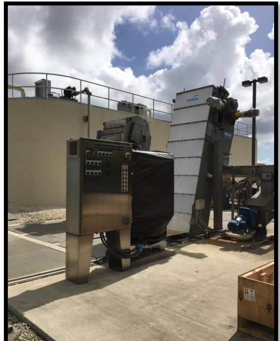
Mechanical Bar screen with new control panel
