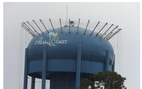
Palm Coast Water Storage Tank Restoration in progress.
