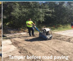
Stormwater pipe replacement – Ferndale Lane
