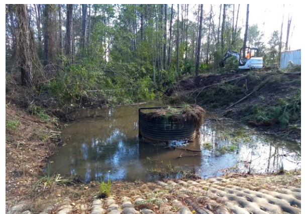
L-1 Surface Water Control Structure
