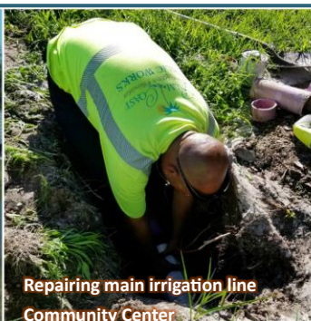
Repairing irrigation -Town Center
