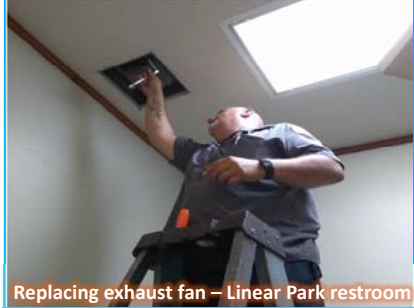
Replacing exhaust fan – Linear Park restroom
