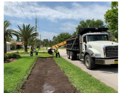
Swale Maintenance - P Section
