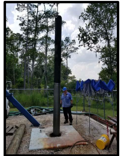
Removing Casing and Well Screen
