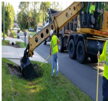
Swale Maintenance - Pritchard drive
