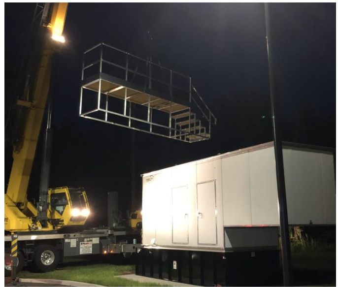
Installing the new generator at the Community Center
