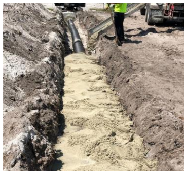
Backfilling Pipe Installation
