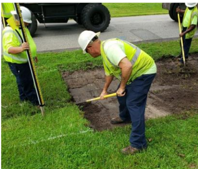
Swale Grading K Section
