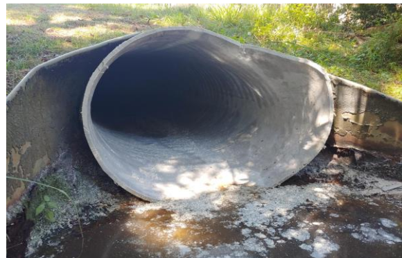
Pipe Lining -P section -after
