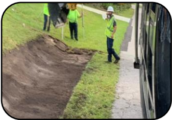
Swale Grading S Section
