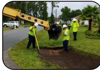
Swale Grading S Section
