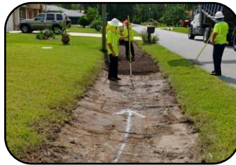
Backfilling Low Swale E Section
