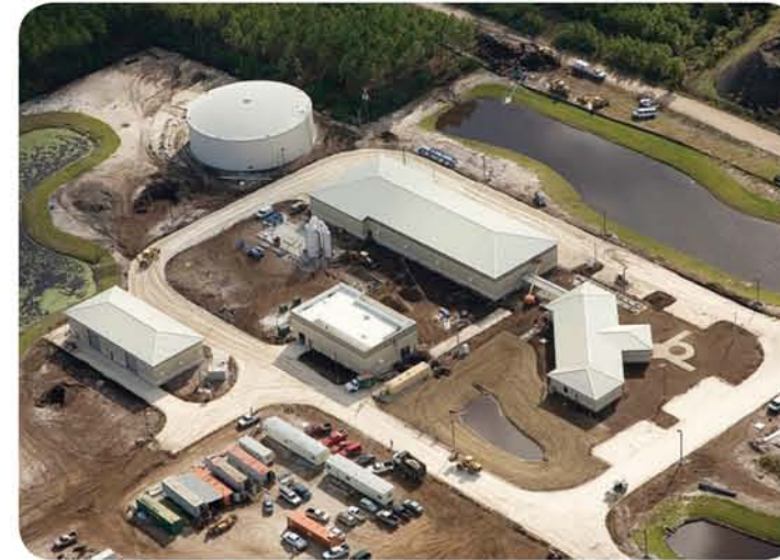
Water Plant No. 3
