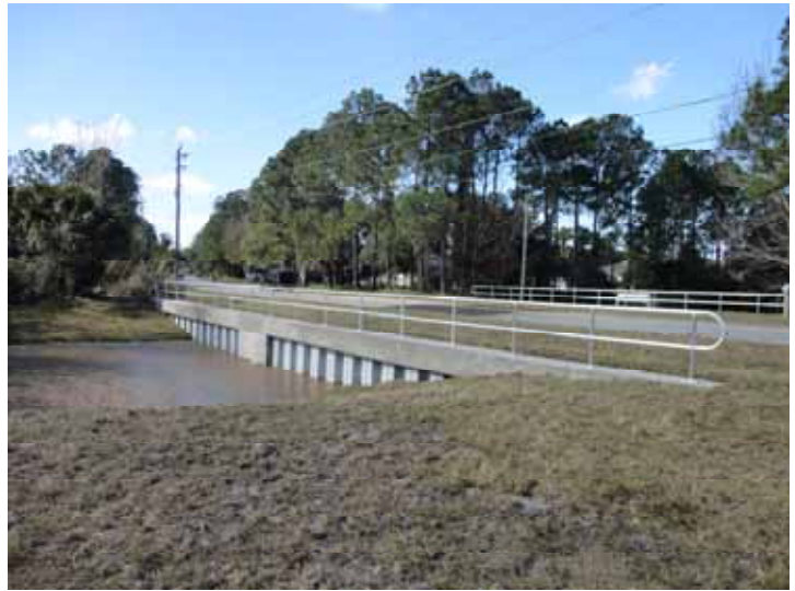
BT-2 After Construction
