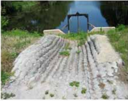
BT - 2 Weir inlet (underwater, upstream)
