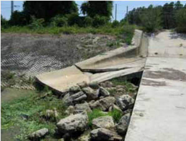
L-4 Weir Before
