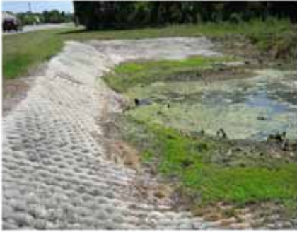
BT - 2 Weir outlet (downstream)
