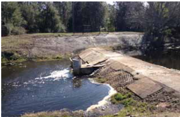
M-3 Before Construction
