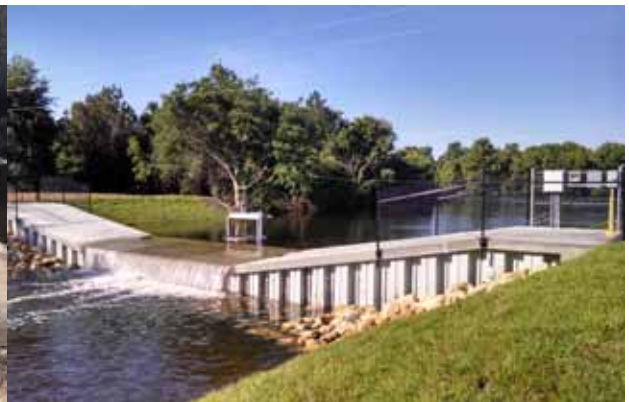
M-3 After Construction
