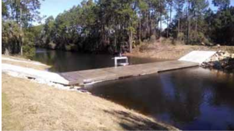
LO-1 Surface Water Control Structure – Completed on March 3, 2015
