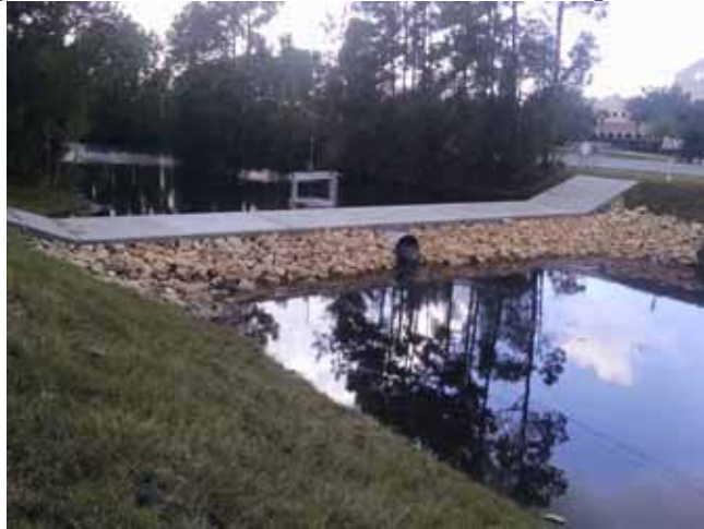
PA-1 Surface Water Control Structure – Completed July 2015
