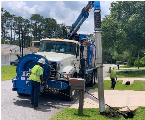
Vac Con Culvert Maintenance – Woodhaven Drive
