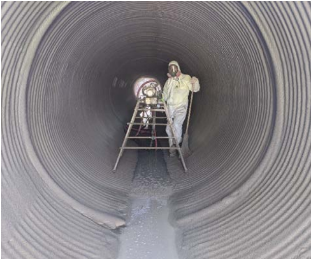
Pipe Lining Activity Enhanced Stormwater Management Program
